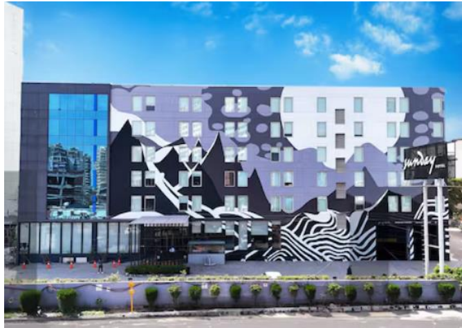
Figure 13: Sunday, Zirakpur Façade
