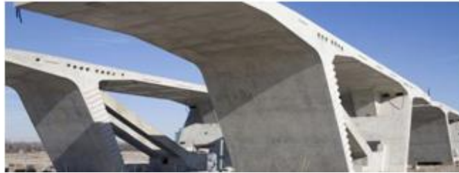
Fig 15) image showing a concrete structure
