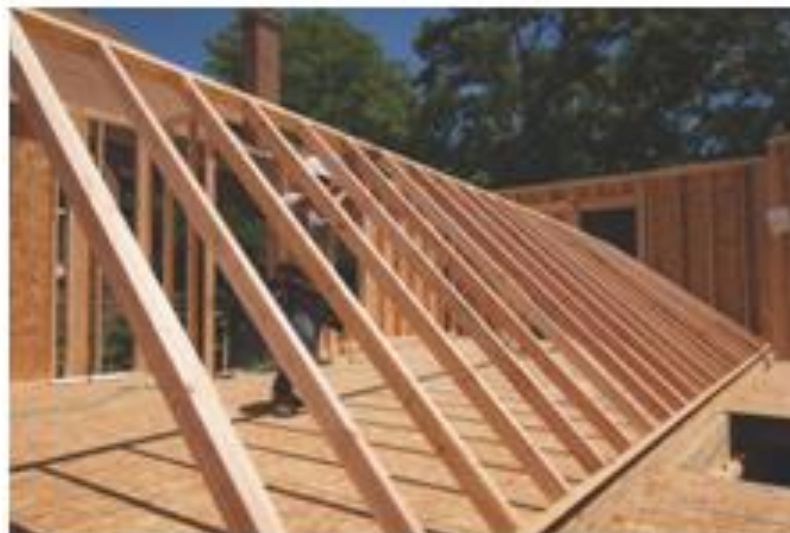
Fig 12) image showing a panelized wood frame
