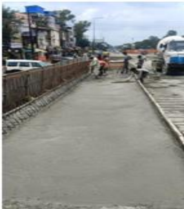
Fig 20) showing stage 2 of construction
