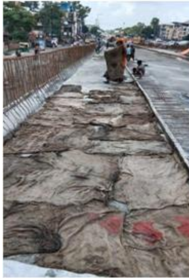
Fig 21) showing stage 3 of construction
