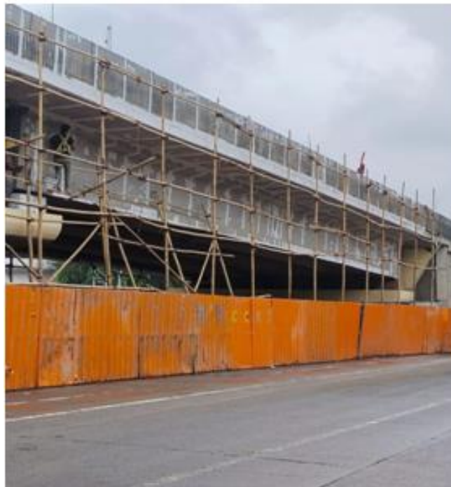
Fig 22) showing stage 4 of construction
