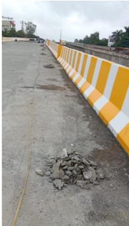
Fig 23) showing stage 5 of construction
