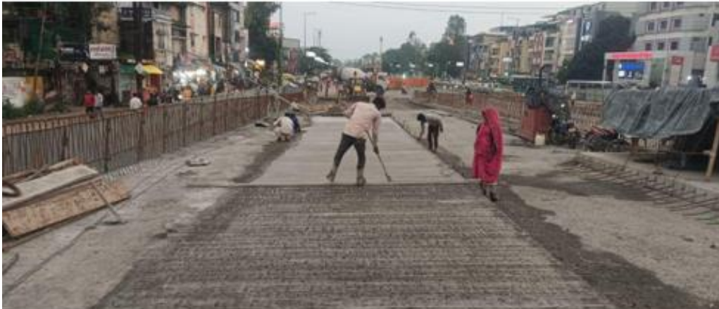
Fig 19) showing stage 1 of construction
