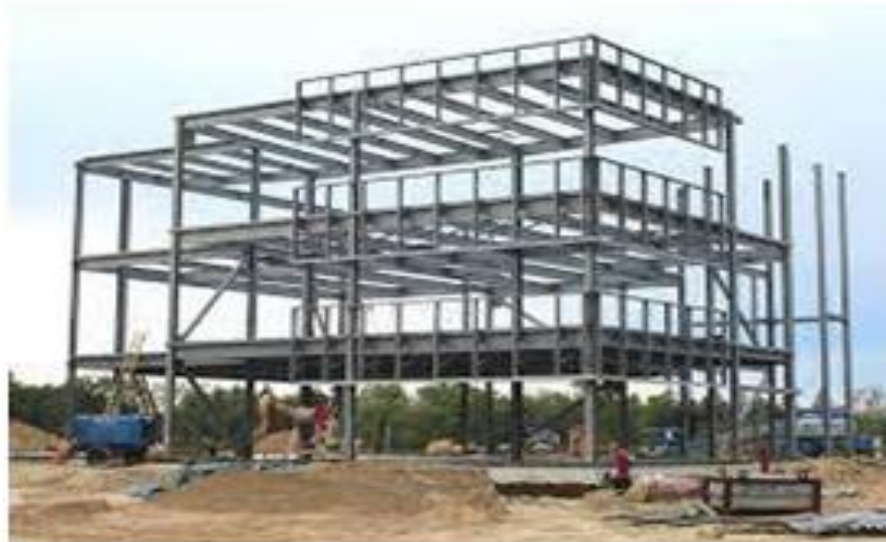
Fig 14) Image showing the building of a steel frame
